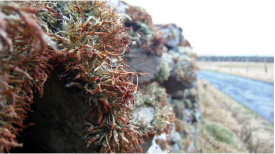
Photo 2. Close-up of Storm-damaged Ramalina siliquosa , west-facing wall, Fair Isle, 8 th February 2017. Photo © Camila Quinteros Peñafiel.
