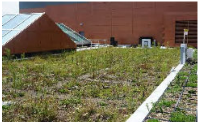
Figure 3. The 24 m x 9 m green roof on the Atrium Building of Saint Mary's University with moveable trays of soil on the right hand (northern) side (photo: Anwar Tumor).
