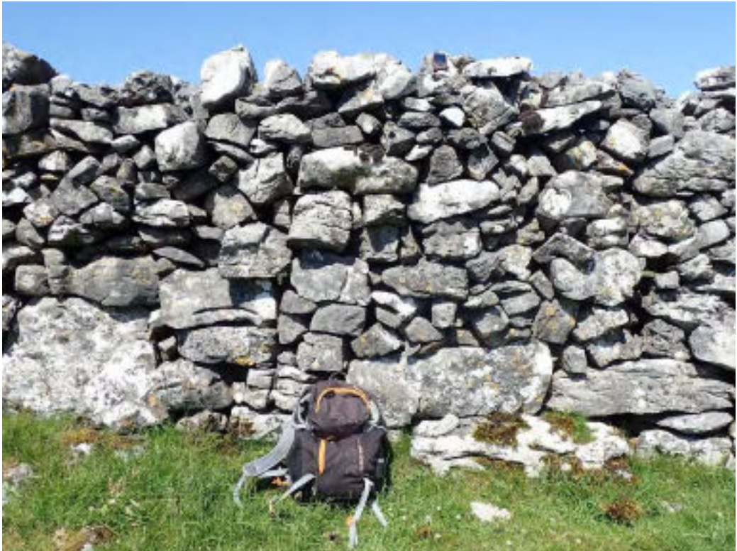
Figure 4. Wall 3. Note the large slabs set on edge at the base of the wall, a characteristic of medieval dry-stone walls (Lord, 2004).
